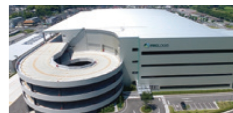
M-30 | Prologis Park Higashimatsuyama JPY 12,600 million
