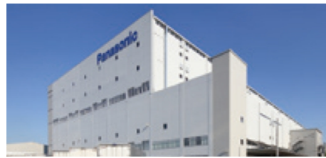
M-014 | Prologis Park Amagasaki 1 JPY 17,600 million
