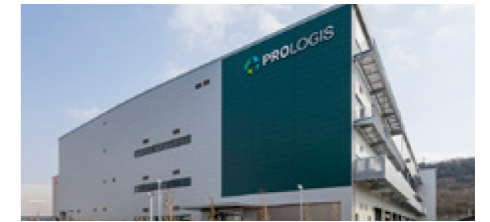
M-37 | Prologis Park Kobe 5 JPY 9,500 million
