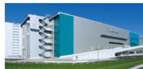
M-29 | Prologis Park Yoshimi JPY 21,300 million
