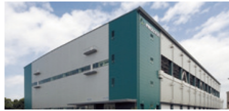
M-07 | Prologis Park Kitanagoya JPY 6,500 million
