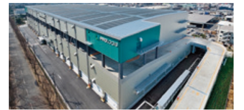
M-25 | Prologis Park Narashino 5 JPY 13,600 million
