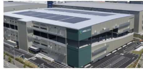
M-39 | Prologis Park Kobe 3 JPY 9,580 million
