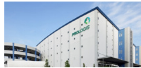
M-15 | Prologis Park Amagasaki 2 JPY 19,200 million
