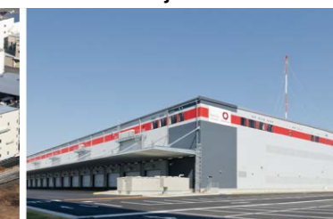
D Project Kuki II
