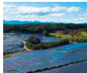
S-10 Takasaki Solar Power Plant A
