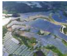
S-01 Takahagi Solar Power Plant
