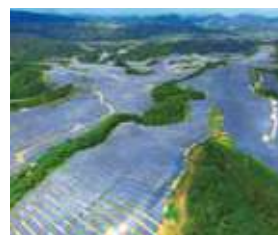
S-07 Matusaka Solar Power Plant
