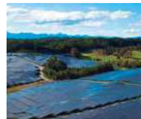
S-10 Takasaki Solar Power Plant A
