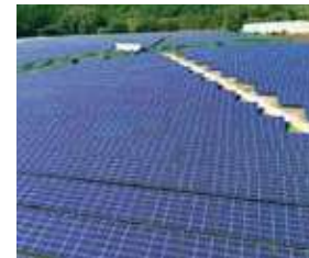
S-05 Hokota Solar Power Plant
