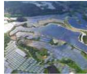
S-01 Takahagi Solar Power Plant
