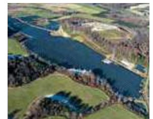
S-09 Monbetsu Solar Power Plant
