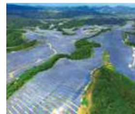
S-07 Matsusaka Solar Power Plant
